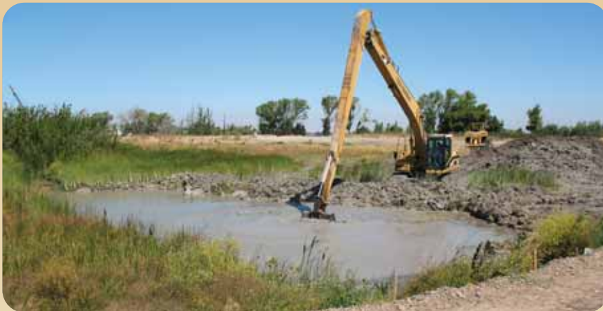
“The Pond” under construction in July 2010.
